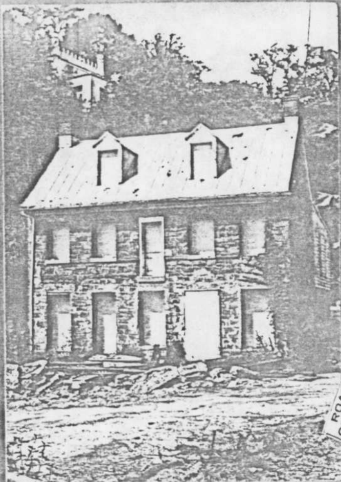
1. Front View (camera facing north)
